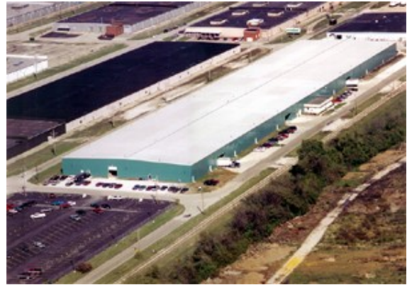
The Everhart Building is adjacent to Fruitridge Avenue with Sony DADC and Bemis as two neighboring industries.
