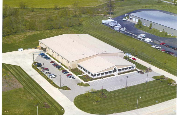
Constructed in 2000, the Doughmakers building is located within the 1,500- acre Vigo County Industrial Park.
